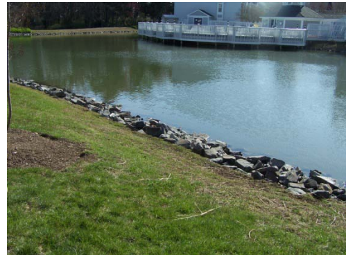
Photo 7 - Riprap section
