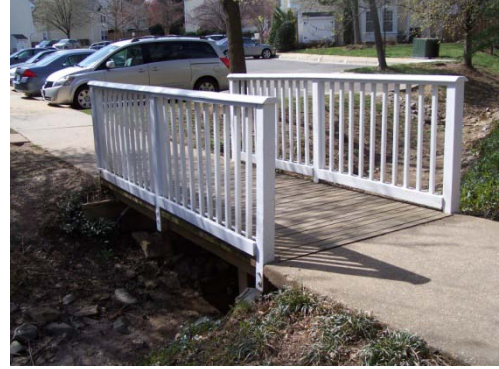
Photo 6 - Wood bridge on path
