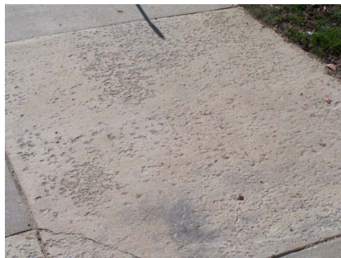
Photo 1 - Spalled sidewalk
