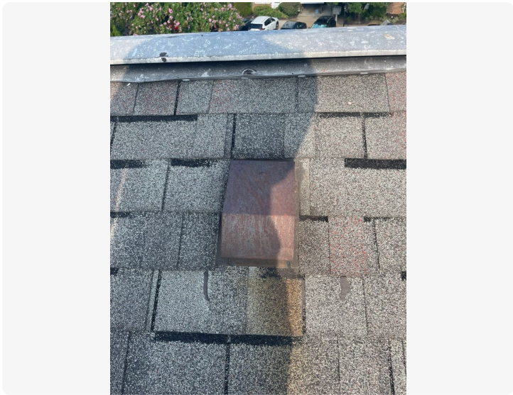
Flashing in good Condition, Vent rusting
