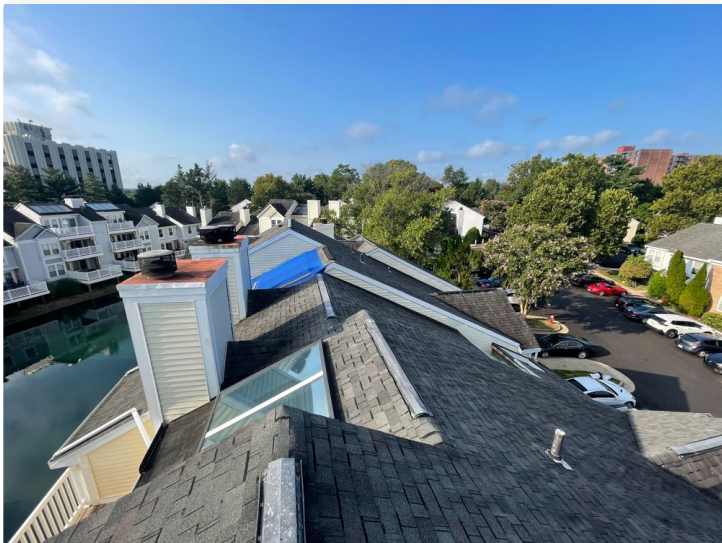
Roof Overview - As Pictured Below
