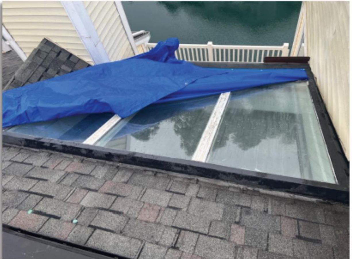
Figure 1: Skylight in Roof over 3311 Lakeside Drive, Bailey's Crossroads, VA 22041 (also known as, Unit 2-6 in Water's Edge Condominium).
